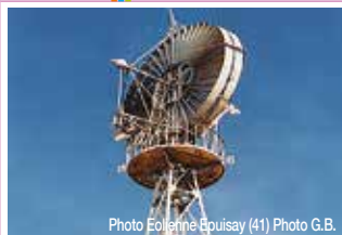
Photo Eolienne Equisay (41) Photo G.B.
